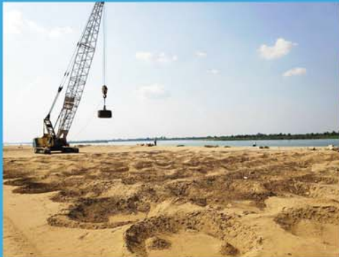
Dynamic Compaction for the Construction of Phase III Container Yard
