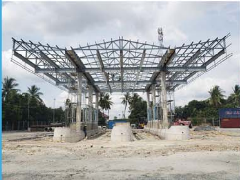
Construction of New Gate
