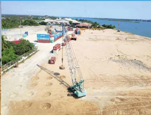
Dynamic Compaction for the Construction of Phase III Container Yard
