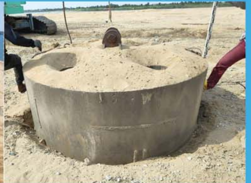
Dynamic Compaction for the Construction of Phase III Container Yard
