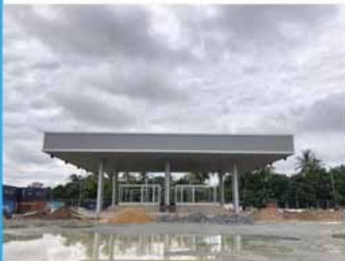
Construction of New Gate
