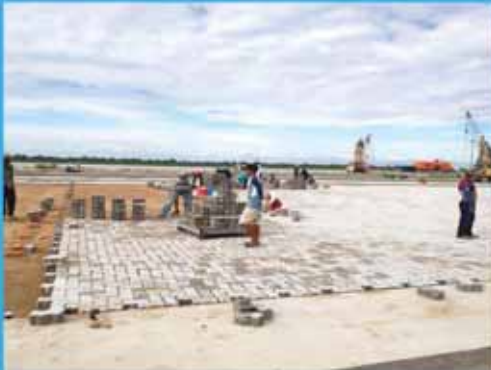
Construction of RTG lanes and concrete block yards for Phase III Expansion of the Container Yard.
