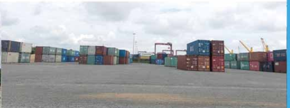
Construction of 3 hectares of Inland Container Depot (ICD)
