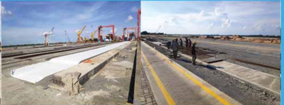
Construction of RTG lanes and concrete block yards for Phase III Expansion of the Container Yard.
